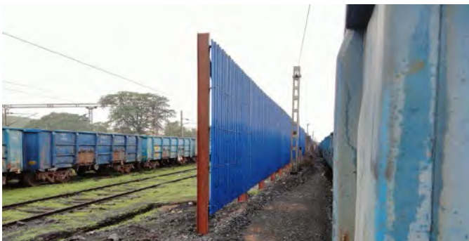
Wind Breaking system at Piparwar & RCM Railway Siding of Piparwar Area
