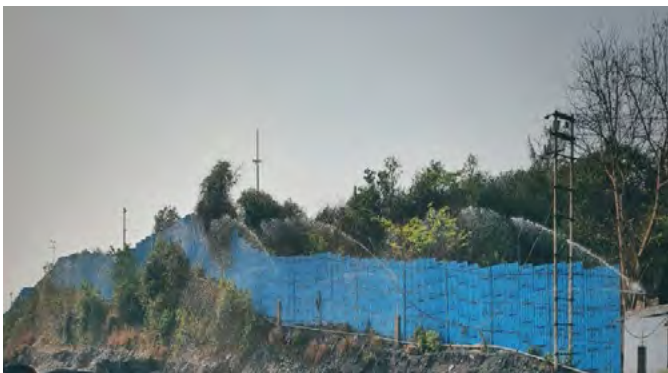
Wind Breaking system at Tarmi Railway Siding of Dhori Area
