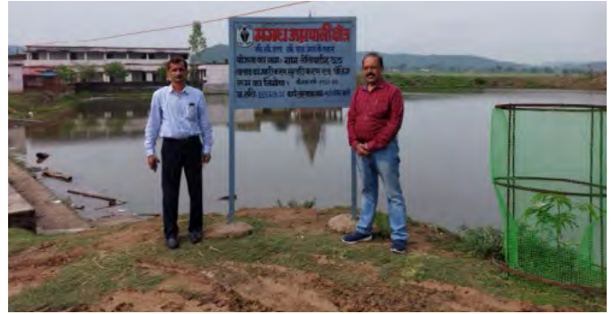
Construction of Pond, Teliyadh, M&A Area
