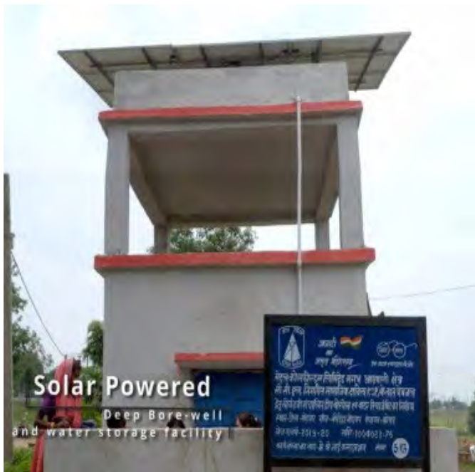
Solar Power operated Deep Bore well
