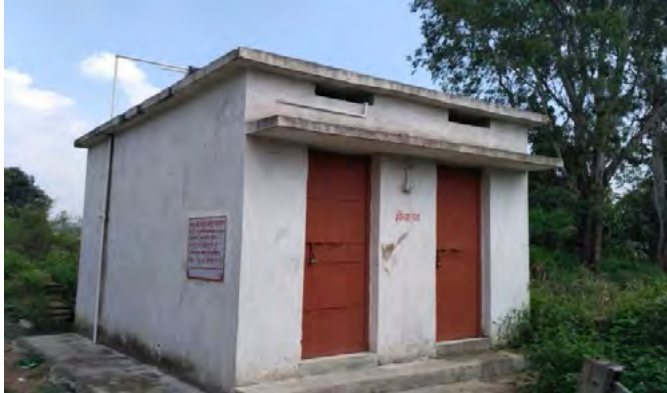
Toilet Constructed under CSR
