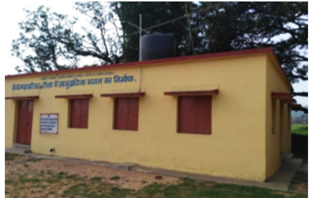
Construction of Community Hall at Hendegarha (Hazaribagh) under CSR
