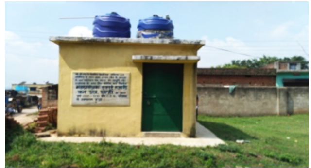
Community Toilet at Hazaribagh Area
