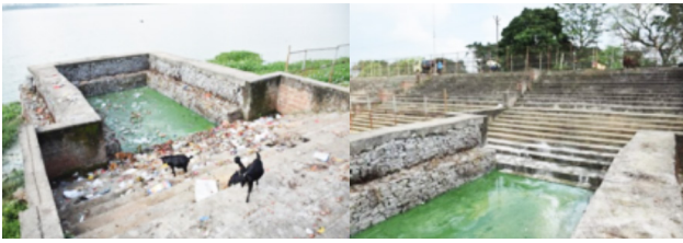
Cleaning of Kanke Dam Reservoir during Swachhta Hi Sewa
