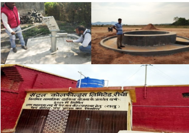
Drinking Water facilities in CCL command area through CSR
