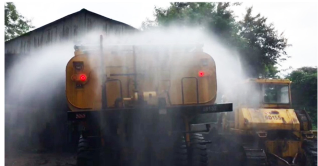
Mist Sprinkler in Operation
